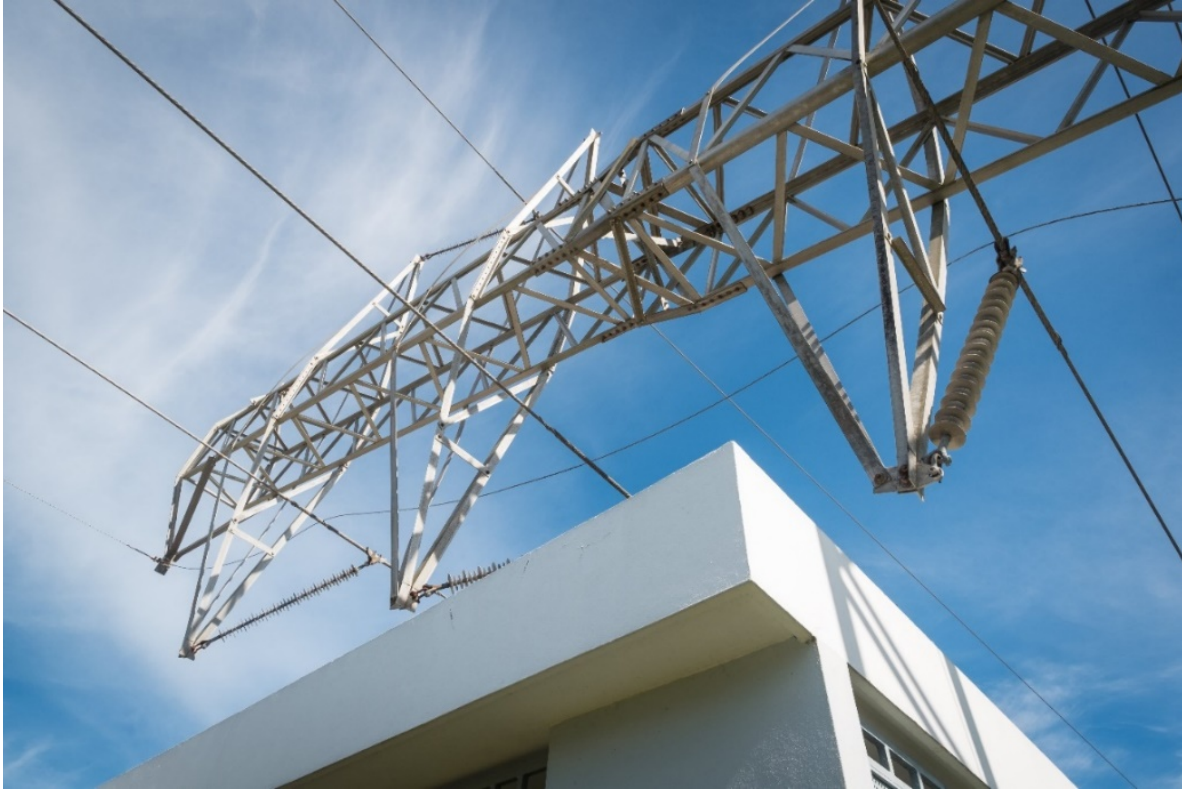
Figure 24 - Guaynabo, Puerto Rico – Power lines remain broken and down along roads and residential areas nearly three months after Hurricane María
