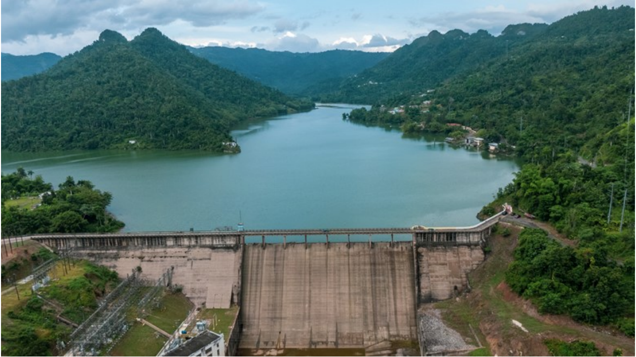
Figure 2 - Dos Bocas Hydroelectric Plant
